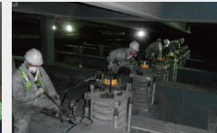
Sling rod balancing
