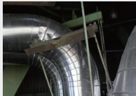
Breakage of Piping support device
